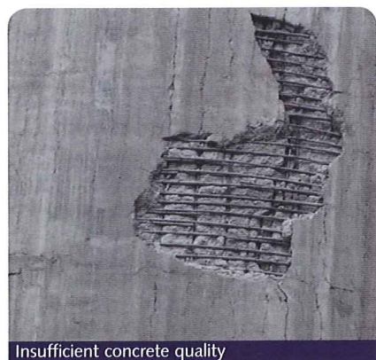
Insufficient rebar cover and concrete quality
